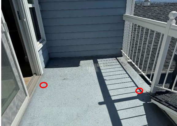
Figure E5 (33665): Drill 1" hole through finish BELOW ledger location and post location at upper deck. Inspection will be provided via endoscope.
