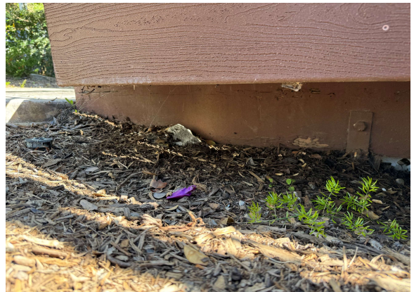
Figure 8: Wood in contact with soil.
